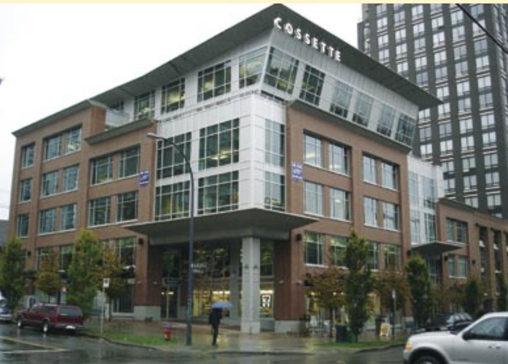
Same property: After recent redevelopment
