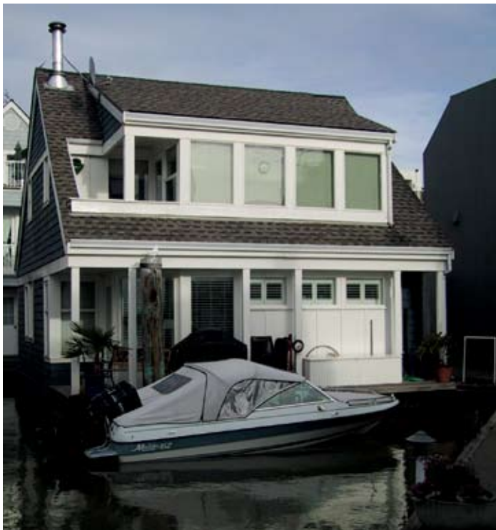
Some float homes include moorage for the owner's boat
