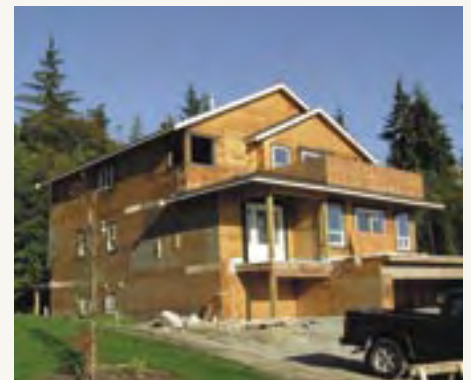
A Neighbour's Home-in-Progress
